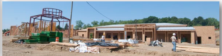
Above: A view from the upper parking lot of the back side of the community center and classrooms with the plywood walls now completed. Left: With the steel completed, workers begin to construct the wooden walls of the church. The green turf is in place to protect the floor from the heavy equipment required to reach the height of the ceilings and the dome. Below: A view from the corner of Babcock and Cumberland of the front of the community center; various construction highlights; the raising of the dome steel ring.
