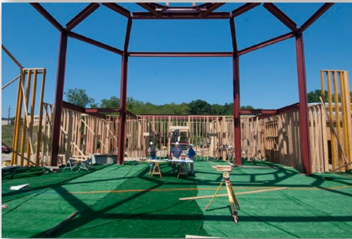
Above: A view from the upper parking lot of the back side of the community center and classrooms with the plywood walls now completed. Left: With the steel completed, workers begin to construct the wooden walls of the church. The green turf is in place to protect the floor from the heavy equipment required to reach the height of the ceilings and the dome. Below: A view from the corner of Babcock and Cumberland of the front of the community center; various construction highlights; the raising of the dome steel ring.
